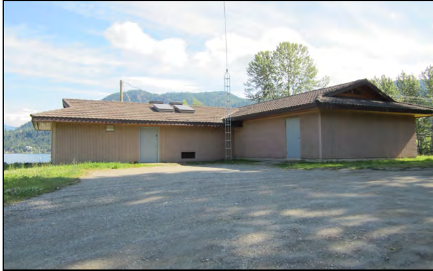
Main pump house - Centennial Drive & Blind Bay Road
