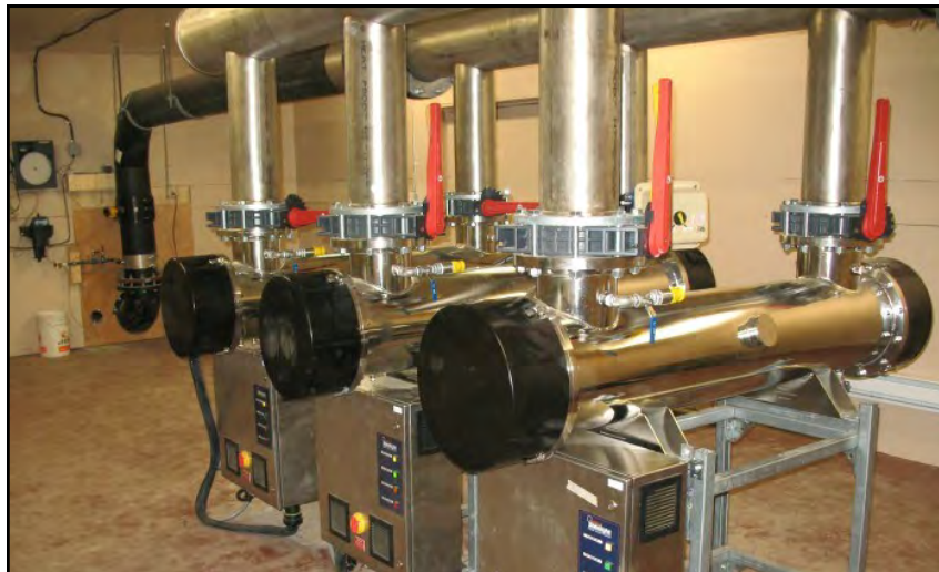
Municipal Sterilight Ultraviolet Disinfection System
