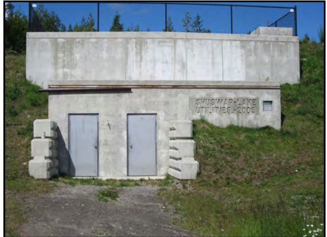
Highlands 1645 reservoir & Chlorine booster station
