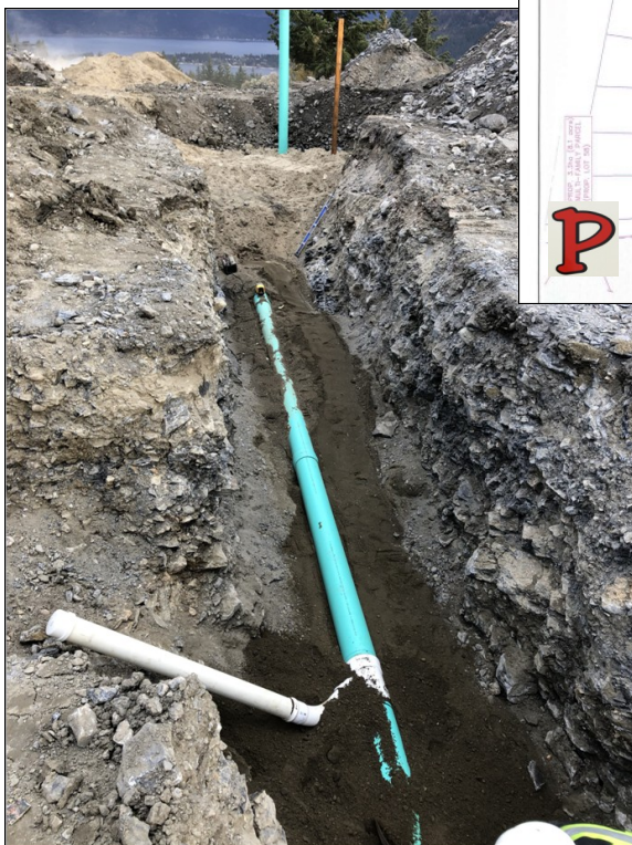
Left, installing the lines.
